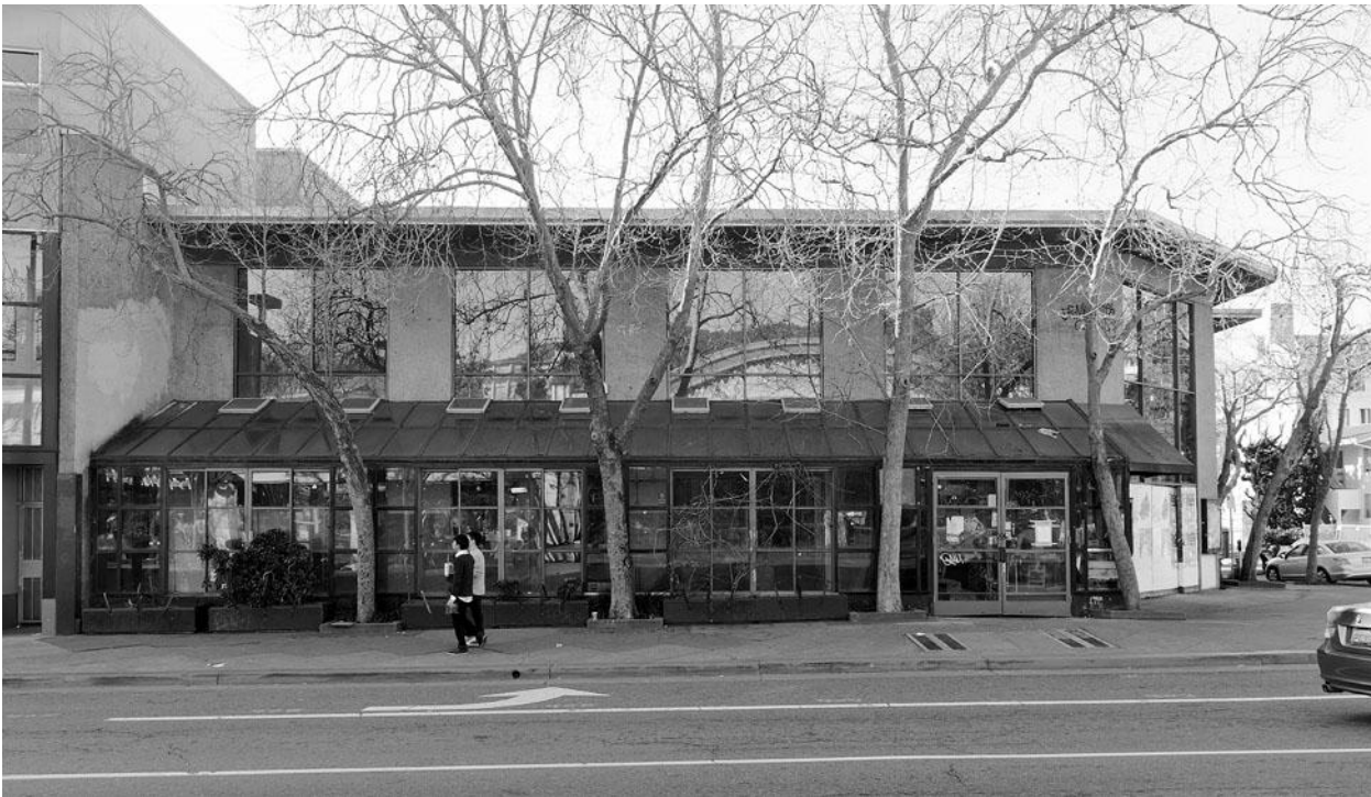
Site View, Telegraph Avenue Frontage
