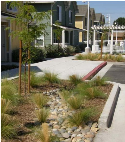
**Vegetated swales (bioswales)** are broad, shallow channels designed to convey and filtrate stormwater runoff.
